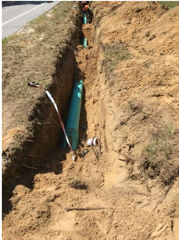
Photo 4: Force main install
