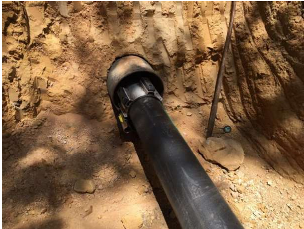
Photo 3: Bore and jack installation
