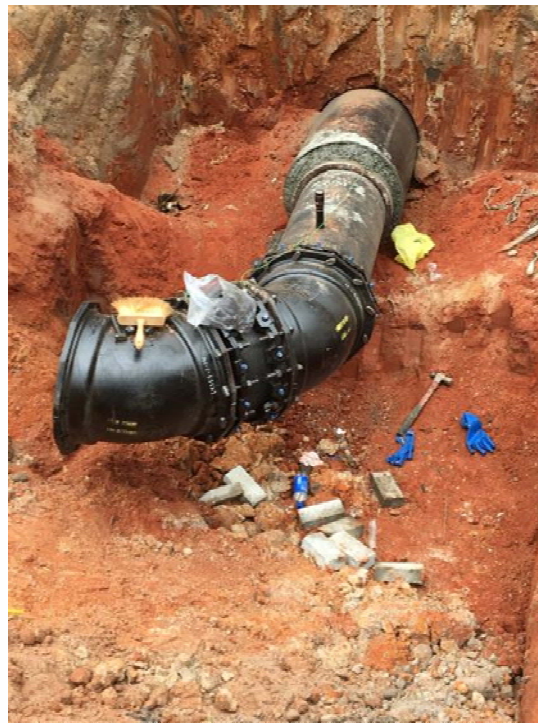
Photo 1: Pipe install in the casing
