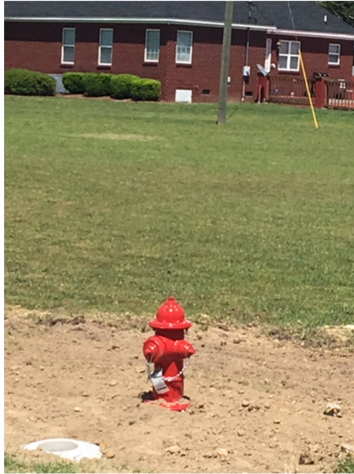
Photo 3: fire hydrant installation on Country Haven Road.
