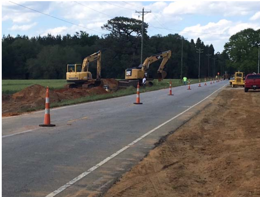
Photo 1: Laying 16” line Lower Richland Blvd
