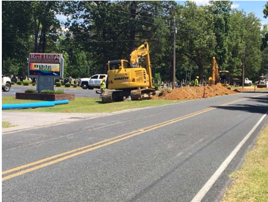
Photo 3: installing water line at Red Hill Church on Congaree Church Road.
