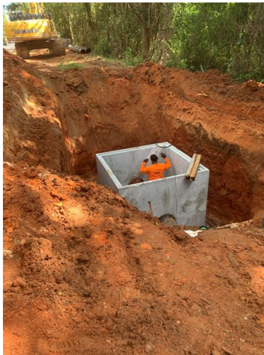
Photo 2: Wet-well install
