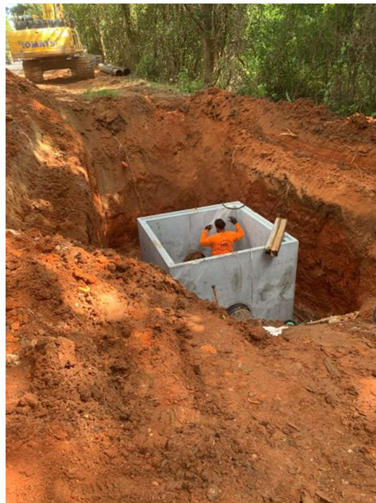
Photo 2: Wet-well install
