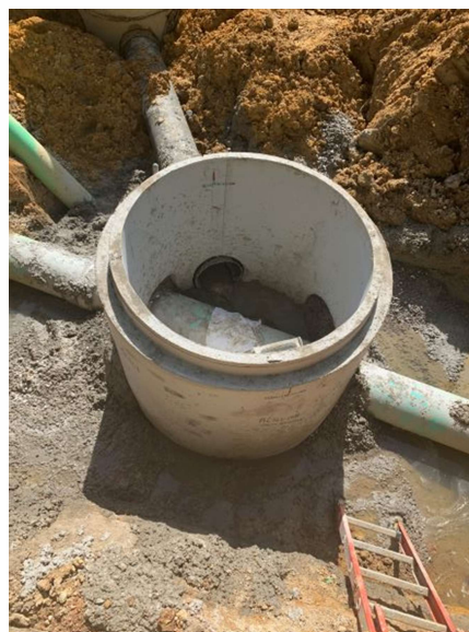
Photo 3: Junction manhole
