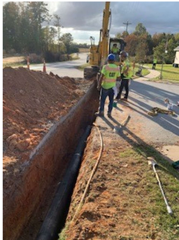
Photo 4: Force main install
