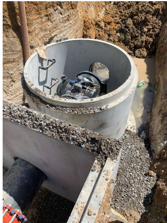
Photo 1: Valve install
