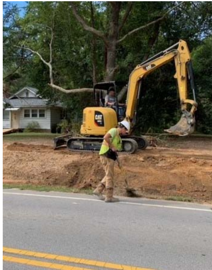
Photo 4: Force main install
