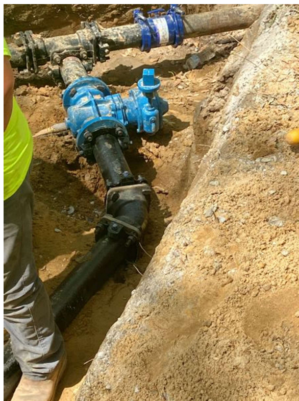
Photo 4: Valve install
