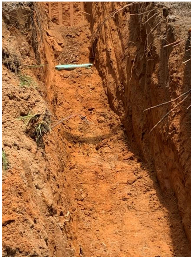
Photo 3: Service connection install
