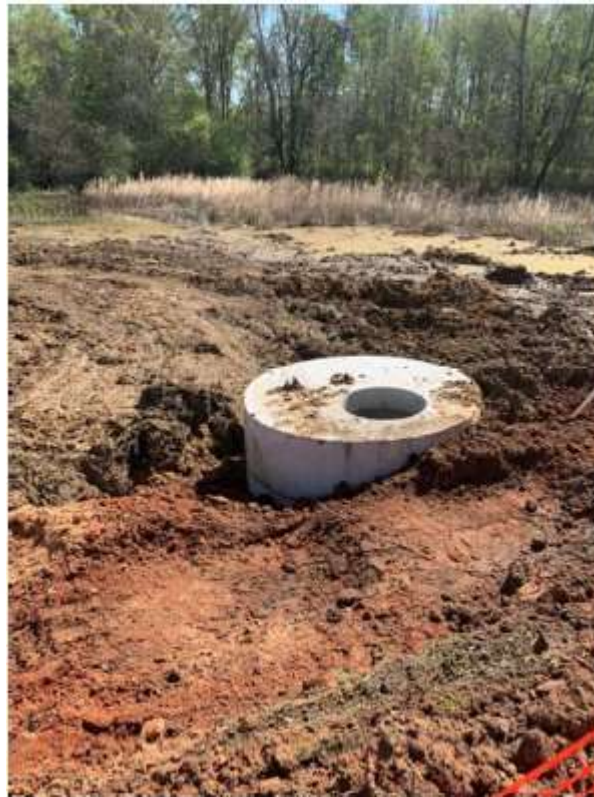
Photo 1: Manhole install
