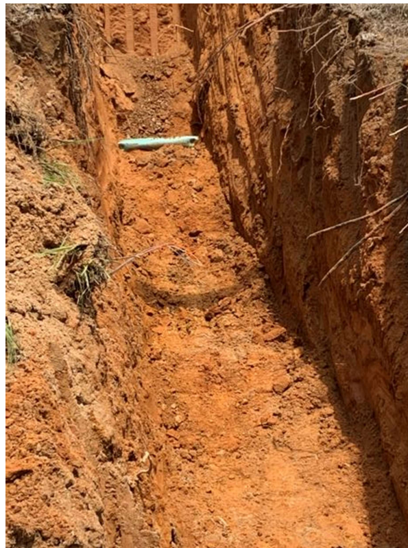
Photo 3: Service connection install
