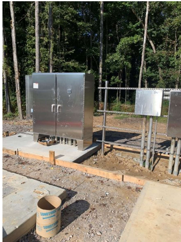
Photo 2: Control panel install
