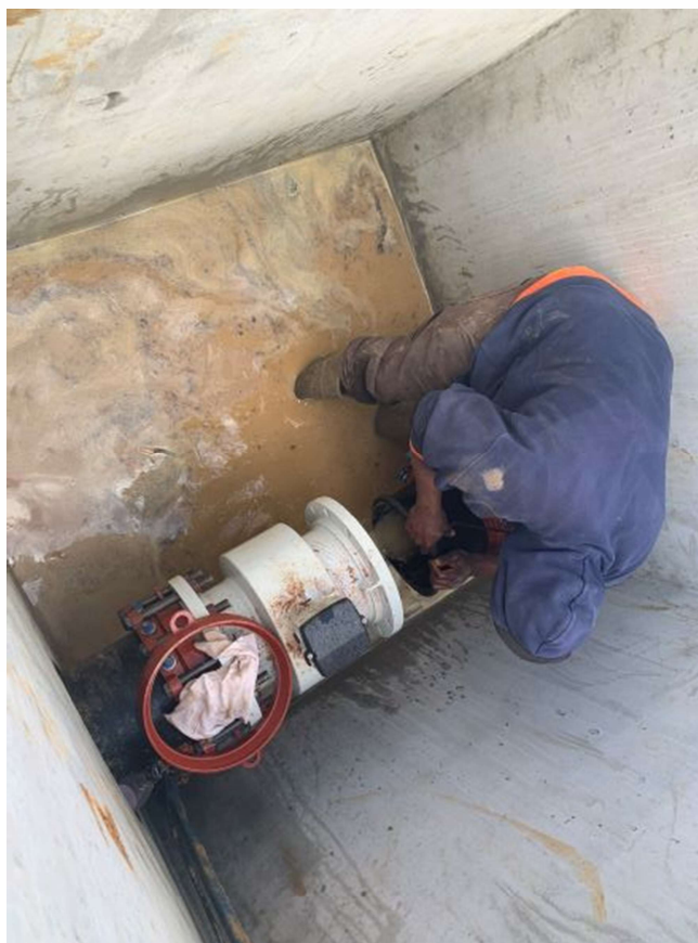
Photo 2: Meter install
