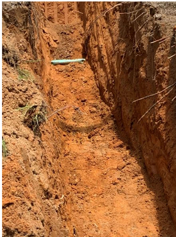
Photo 3: Service connection install
