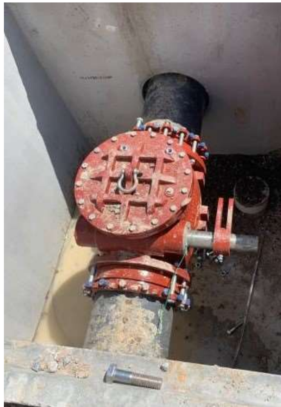
Photo 3: Valve install
