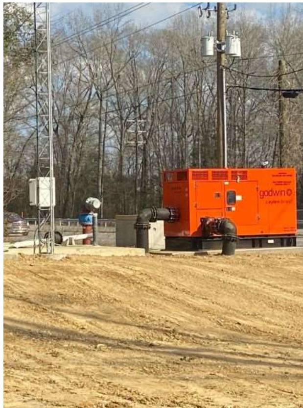
Photo 1: Garners Ferry pump station
