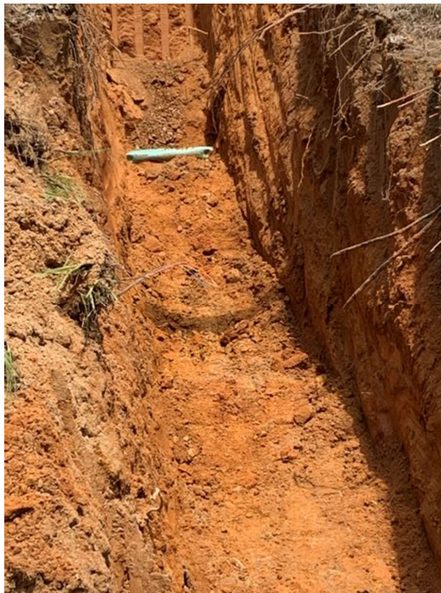
Photo 3: Service connection install
