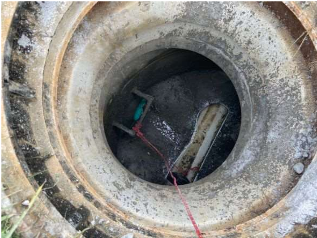
Photo 4: Pump station tie-in
