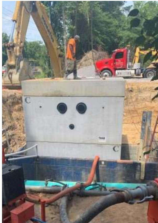
Photo 1: Wet-well install
