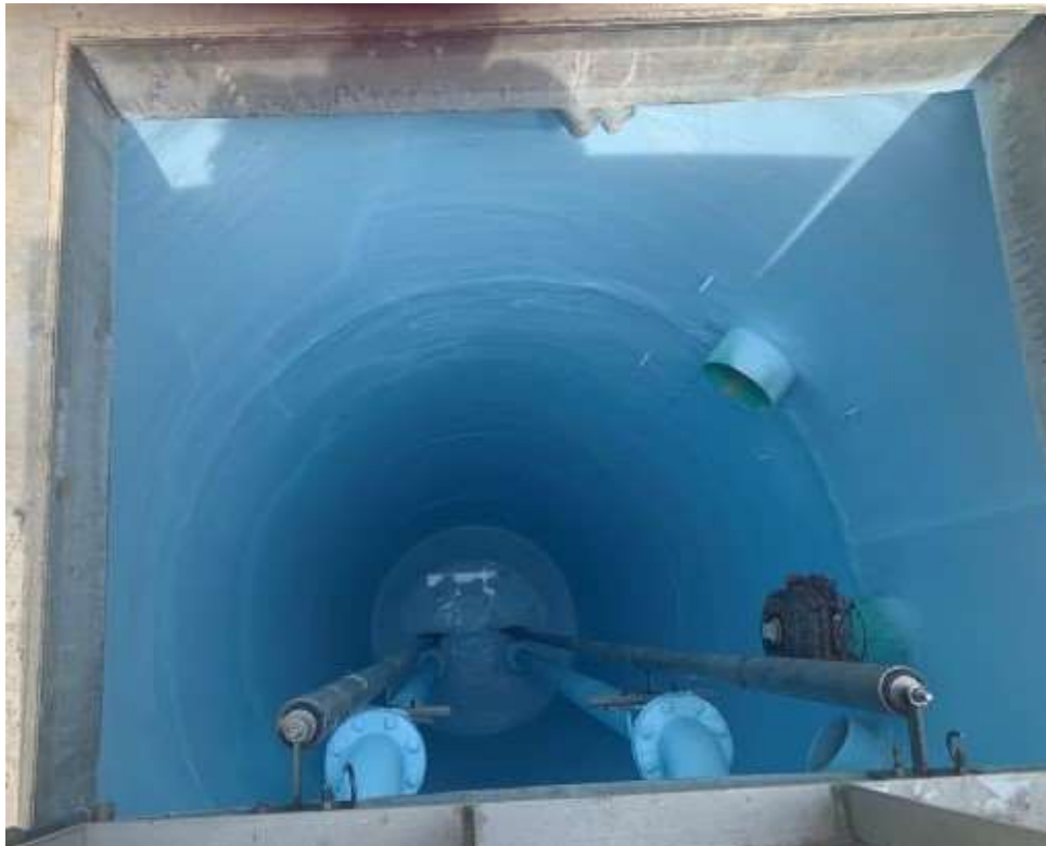
Photo 3: Wet-well Install
