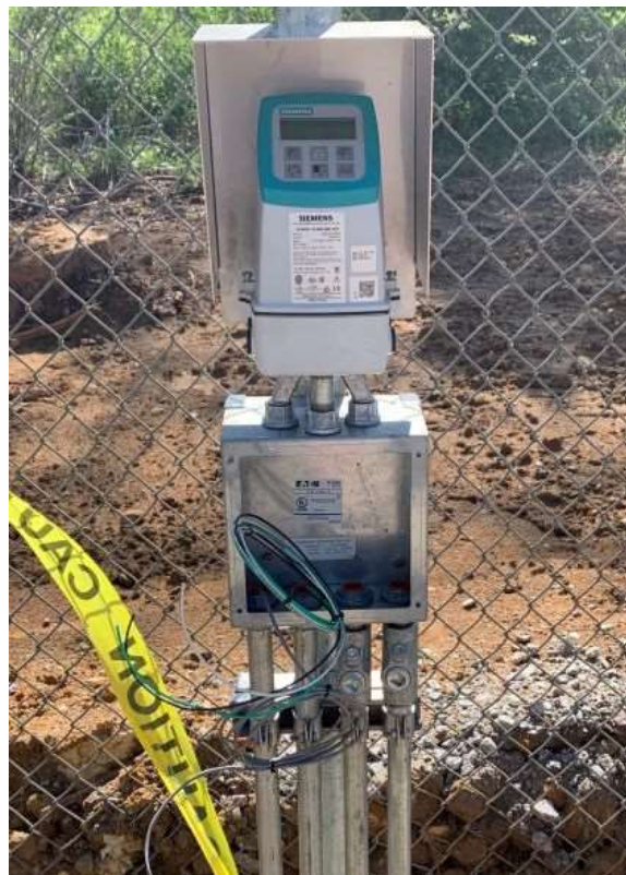
Photo 2: Flowmeter install
