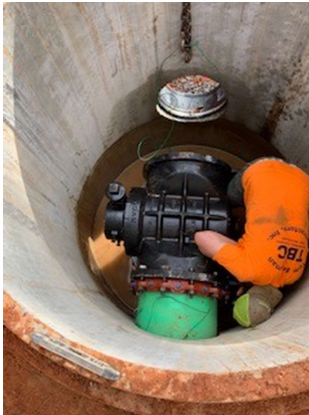
Photo 2: Valve install
