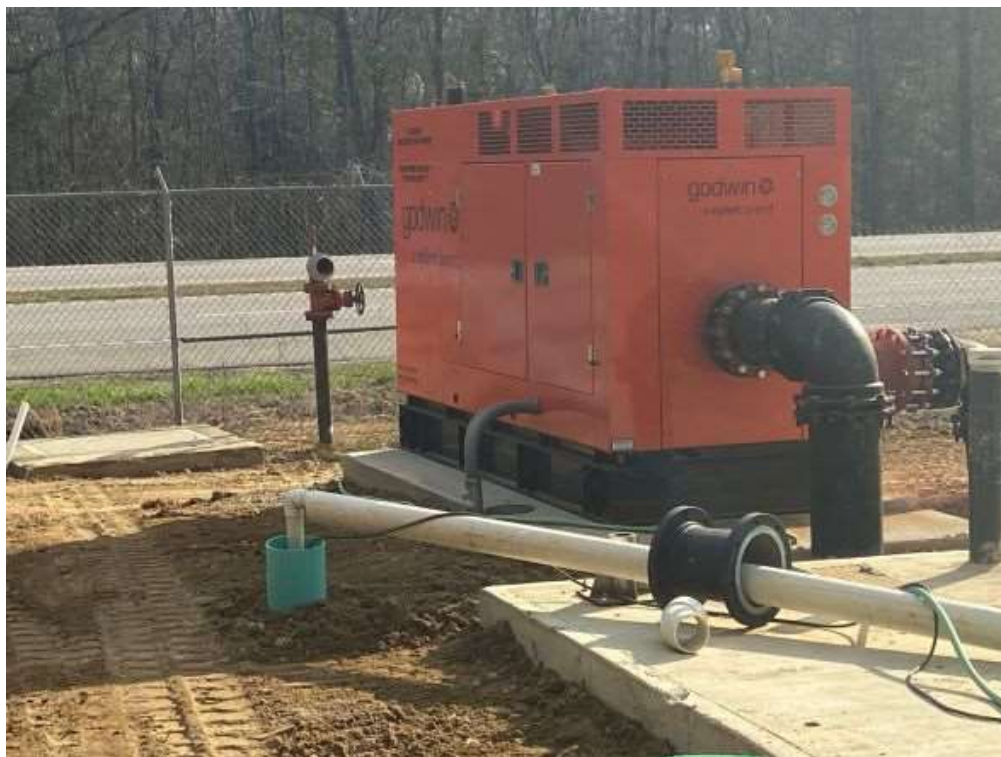
Photo 1: Bypass pump
