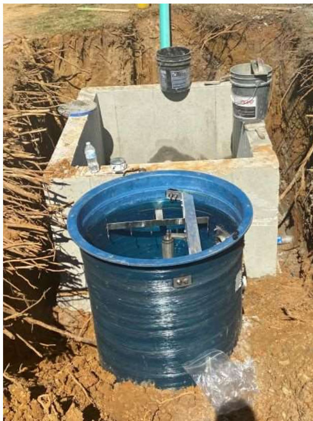
Photo 3: Grinder system install
