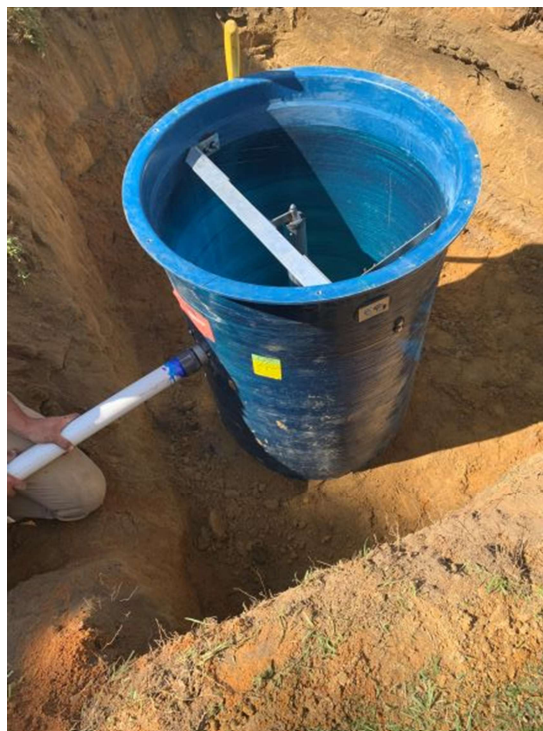
Photo 4: Grinder pump install
