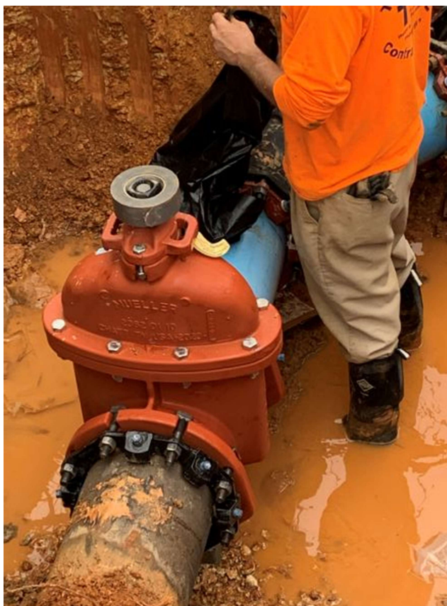
Photo 2: Valve install
