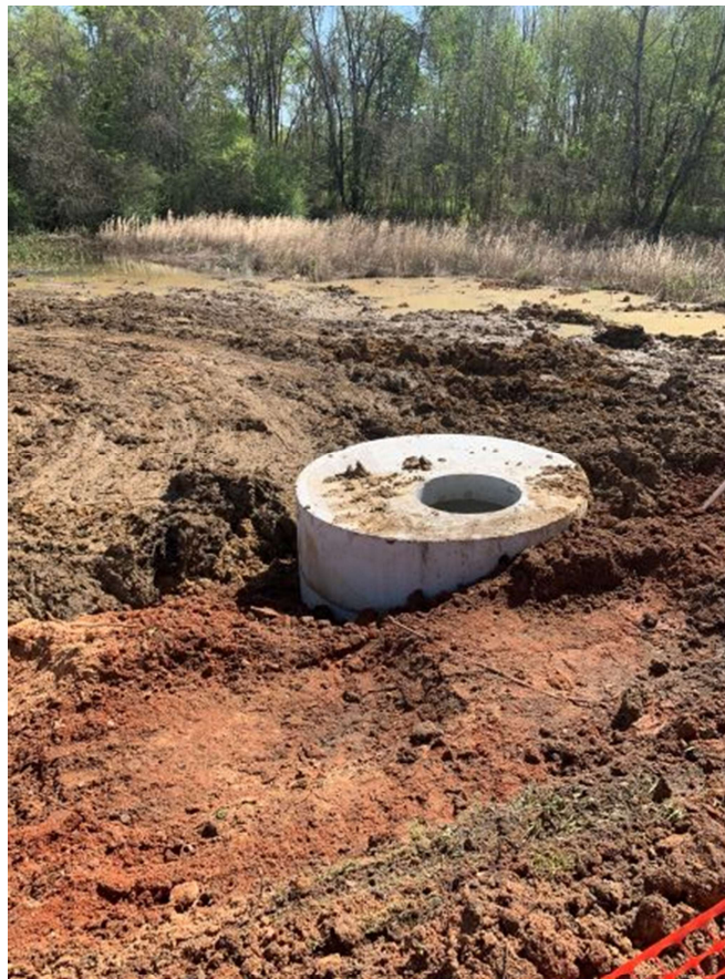
Photo 1: Manhole install
