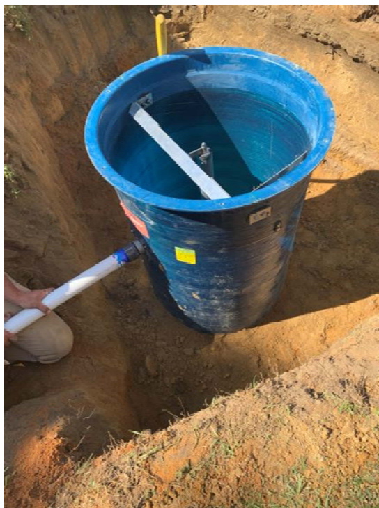
Photo 4: Grinder pump install
