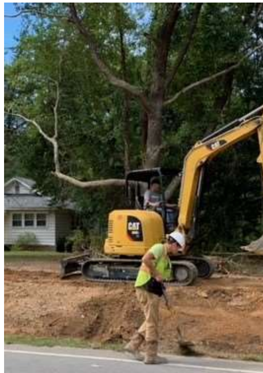
Photo 4: Force main install
