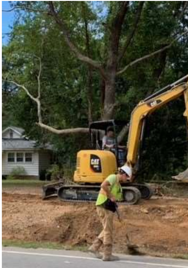
Photo 4: Force main install
