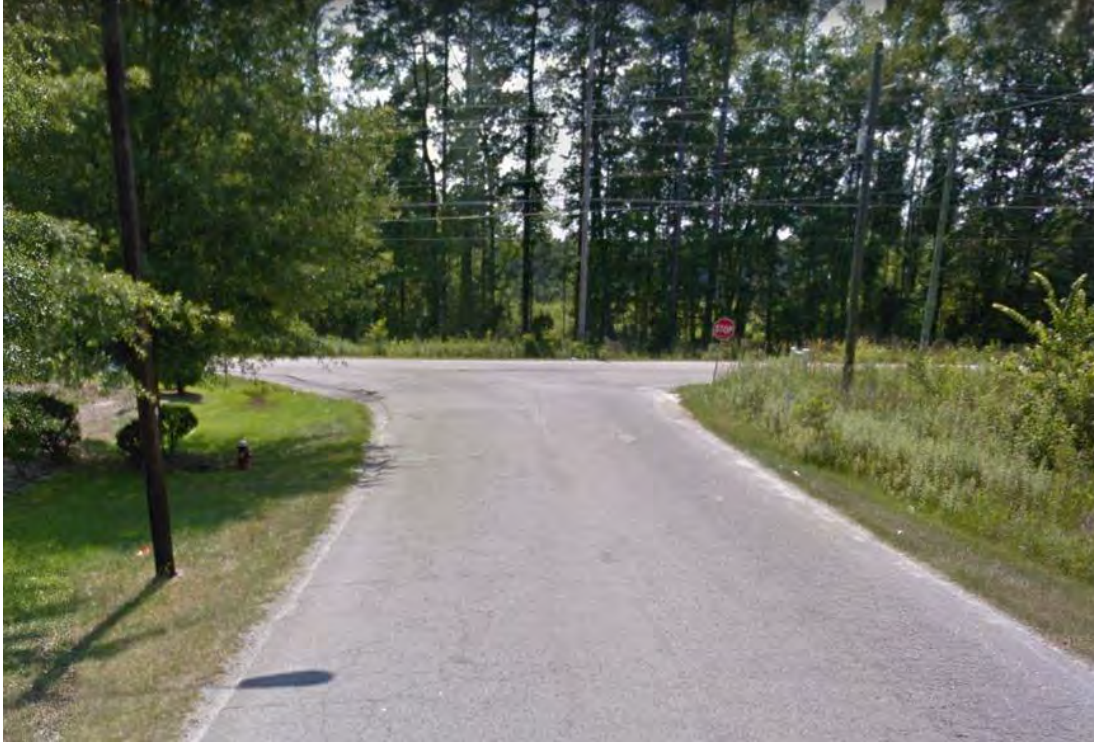
Hobart Road at Farrow Road Intersection
