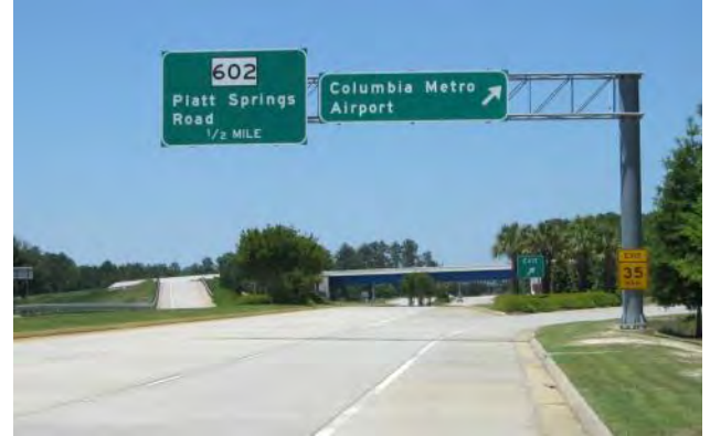
Airport Exit from Phase I of the Airport Connector Project
