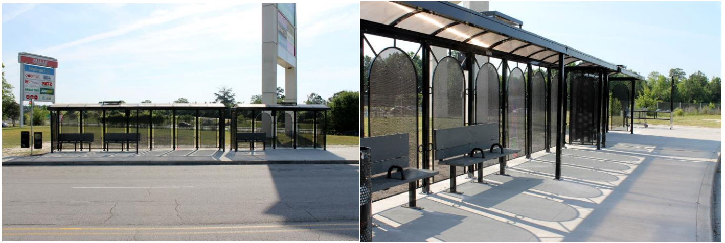
Image 1. Forest Drive Connection Protection Zone
