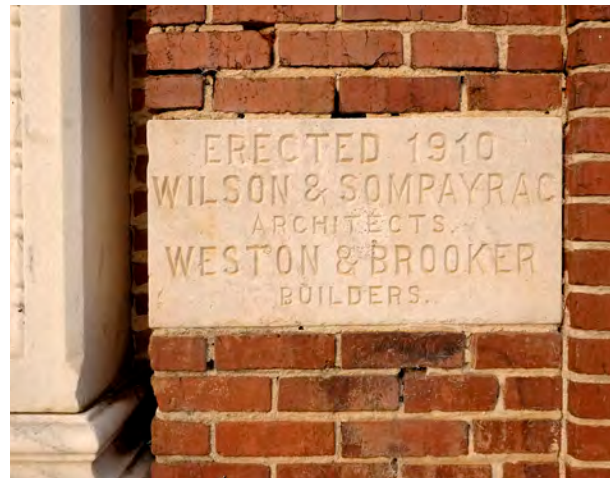
Architectural detail in Eastover
