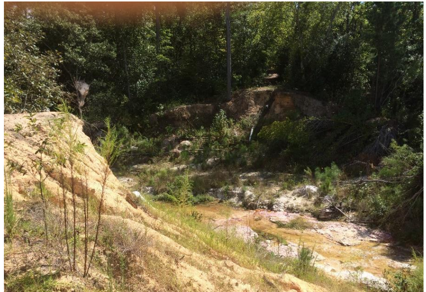
Figure 7. Southeasterly view through dam breach. Note active rilling of northern embankment and sparse vegetation along channel.
