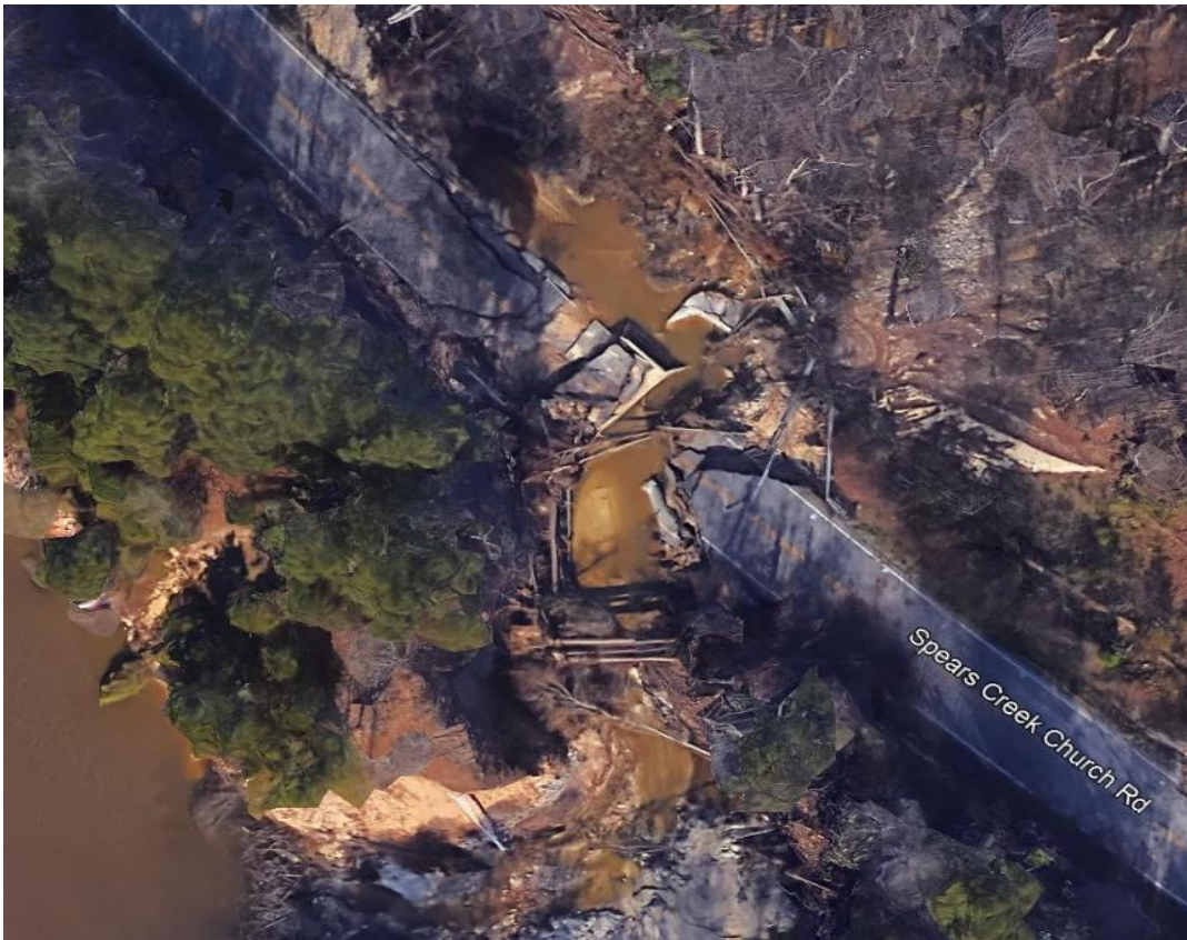
Figure 2. Walden Pond dam breach and road washout after October 2015 floods (Google Earth Pro).
